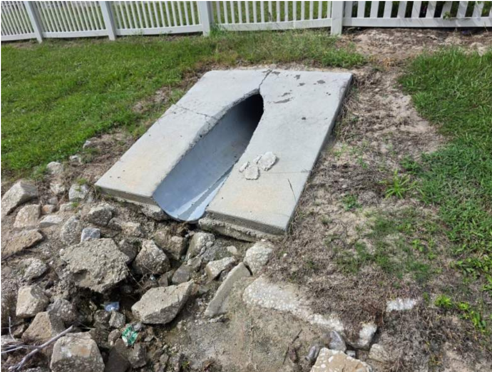
Figure 17. Structure cracking on surface and vegetation reduced around MES. Add soil to restore grade, sod, and monitor.
