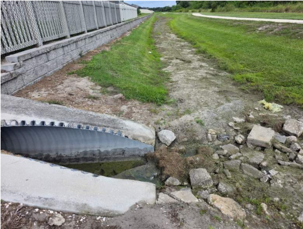
Figure 39. Complete lack of vegetation near MES and retaining wall containing yard drains. Install new sod along structure and wall to prevent further erosion and sedimentation.
