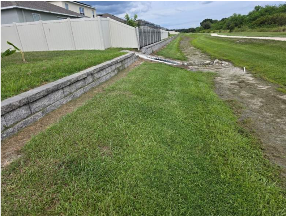
Figure 36. Large patch is bare of vegetation along bank. Add sod and monitor.
