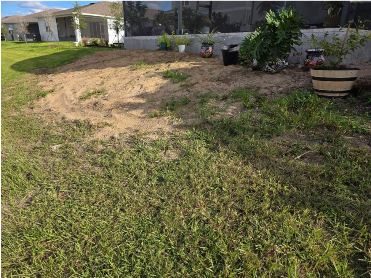
Figure 187. (Figure 187-188) Slope of pond covered in sediment, resident must have excess sediment removed from CDD lands, restore grade, and restore sod if necessary.
