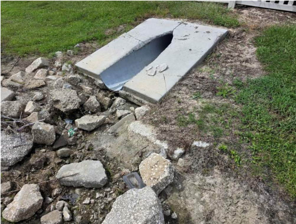
Figure 13. Structure cracking on surface and vegetation reduced around MES. Add soil to restore grade, sod, and monitor.
