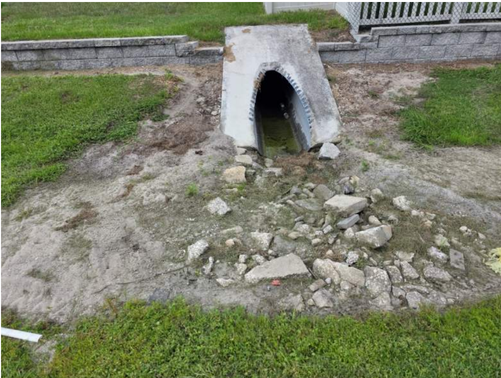
Figure 40. Complete lack of vegetation near MES and retaining wall containing yard drains. Install new sod along structure and wall to prevent further erosion and sedimentation.
