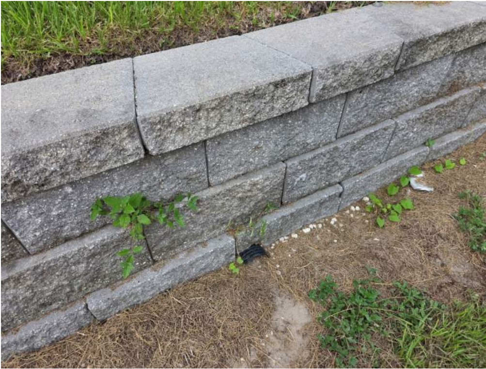
Figure 49. Yard drain blocked with sediment and vegetation. Unclog and monitor.
