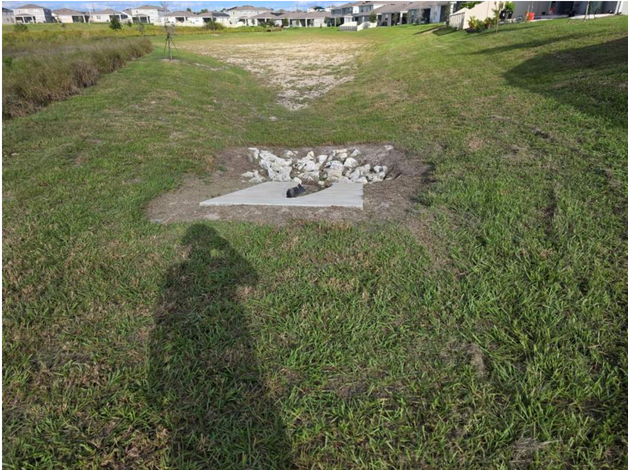
Figure 176. (Figure 176-177) Area around MES lacks vegetative cover, restore grade and sod
