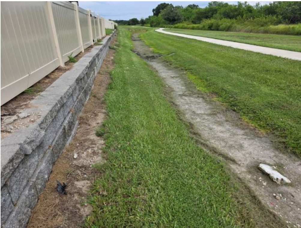
Figure 52. Large patch is bare of vegetation along bank. Add sod and monitor.
