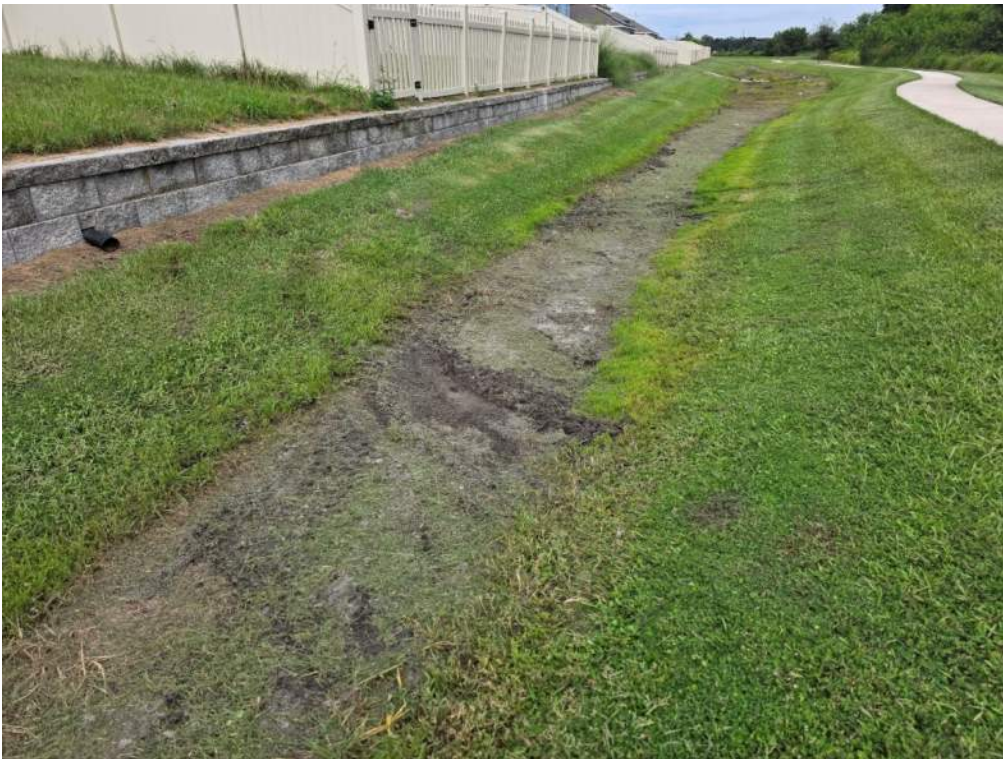
Figure 56. Large patch is bare of vegetation along bank. Add sod and monitor.
