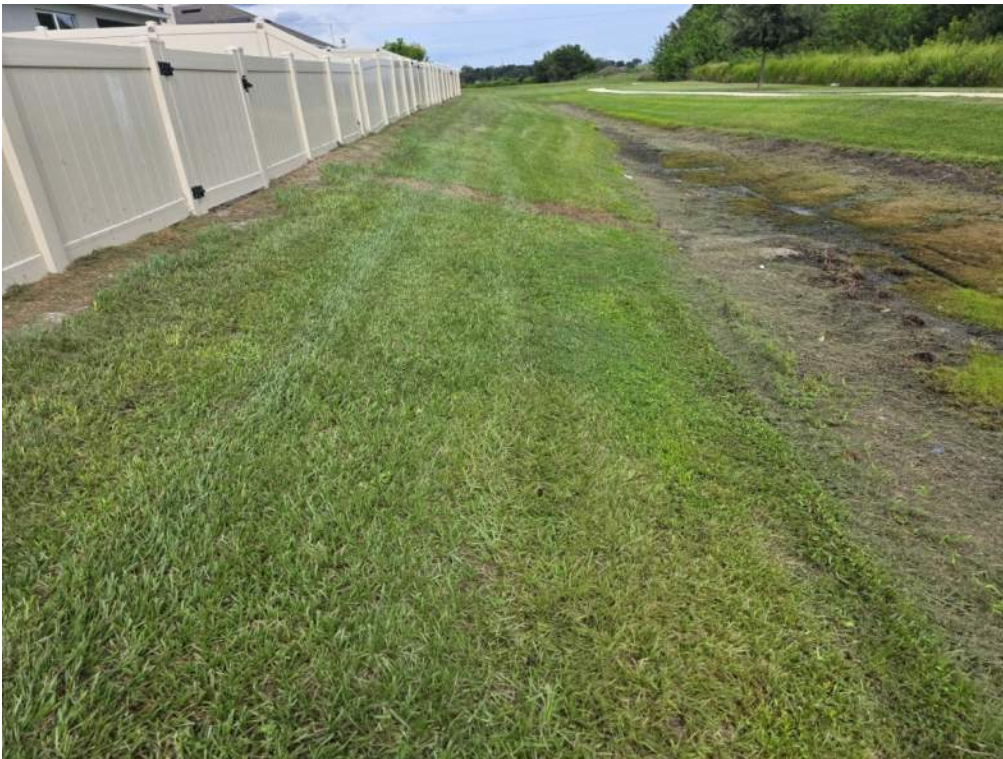
Figure 70. Large patch is bare of vegetation along bank. Add sod and monitor.
