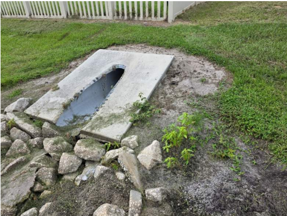
Figure 66. Area around and particularly below MES lacks vegetative cover and soil. Add soil to restore grade and sod. Rearrange riprap after grade restoration and monitor.
