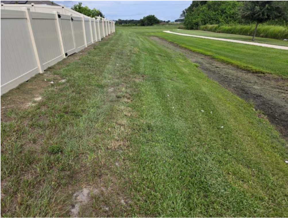
Figure 71. Large patch is bare of vegetation along bank. Add sod and monitor.
