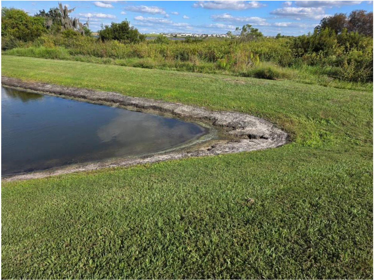
Figure 146. (Figure 146-157) Pond bank lacks vegetative cover, monitor growth and water level
