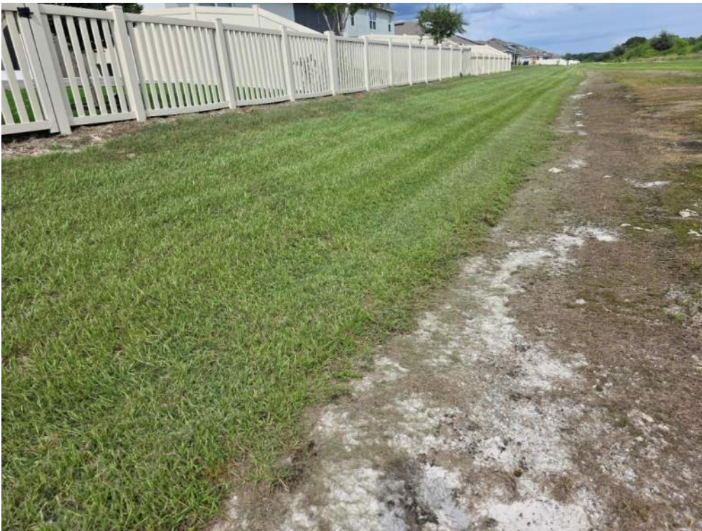
Figure 28. Large patch is bare of vegetation along bank. Add sod and monitor.
