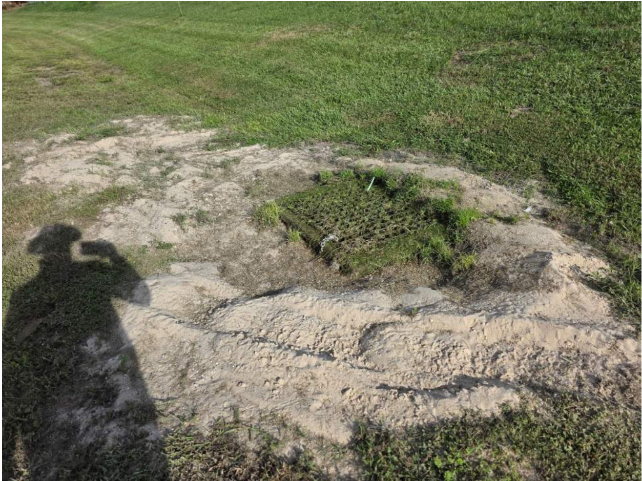
Figure 198. (Figure 198-199) Control structure overgrown and sediment has been piled around structure. Clean off growth and remove sediment to allow for proper drainage.
