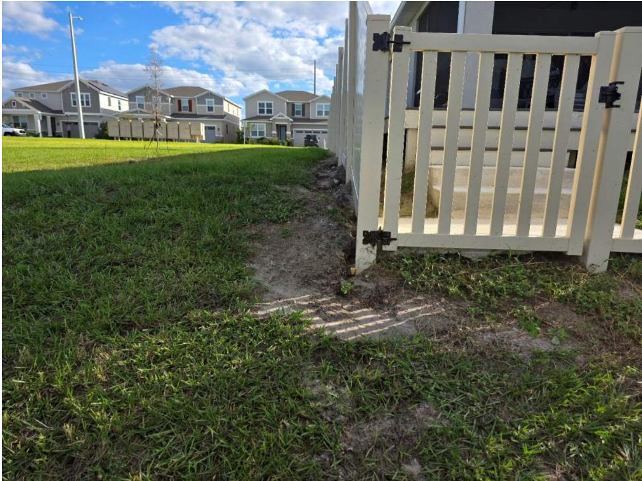
Figure 160. (Figure 160-163) Area lacks vegetative cover, fence post support exposed, reduce herbicide spraying, restore cover, and sod
