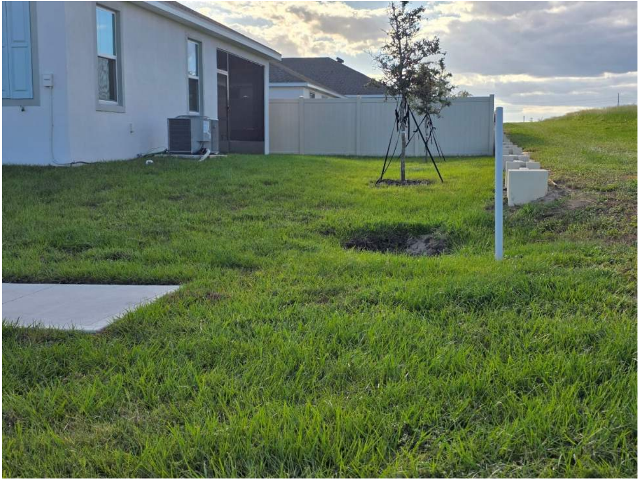
Figure 237. Soften grade to control structure to eliminate trip hazard.
