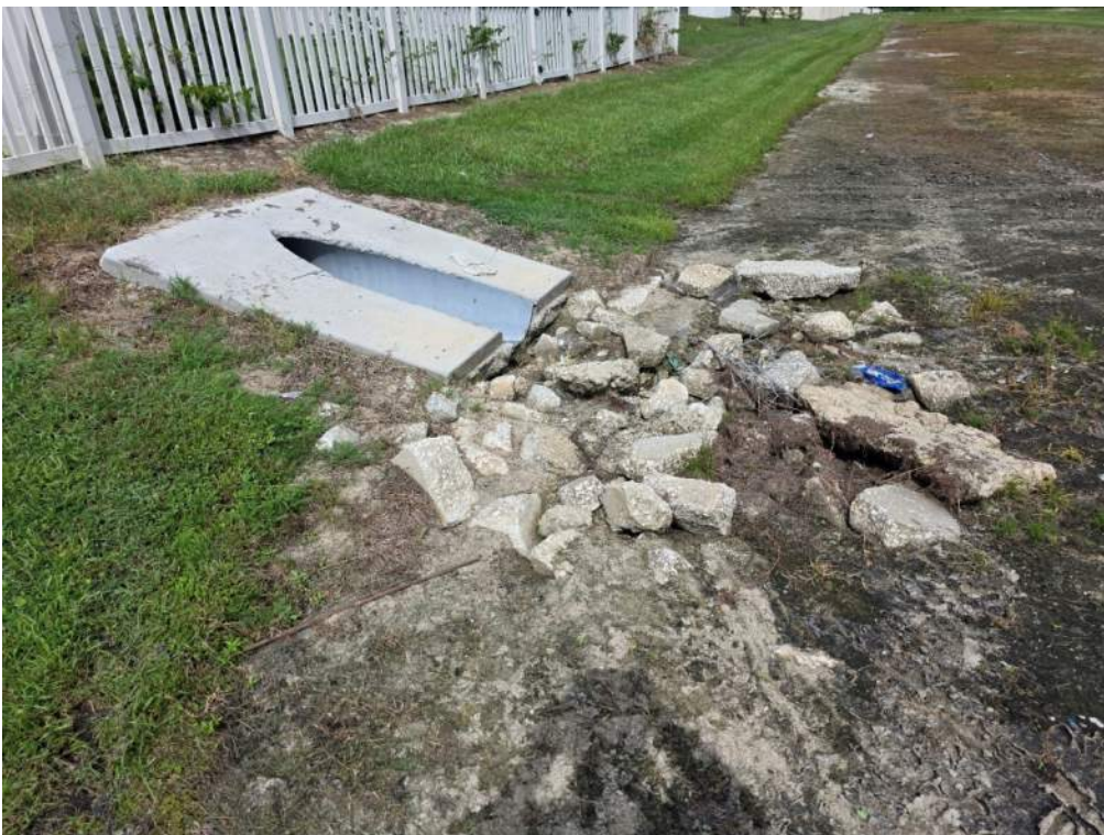
Figure 12. Structure cracking on surface and vegetation reduced around MES. Add soil to restore grade, sod, and monitor.
