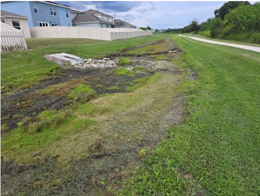
Figure 62. Baseline photo, bottom of pond. No action needed. Deep cuts in soil due to vehicles driving through pond.
