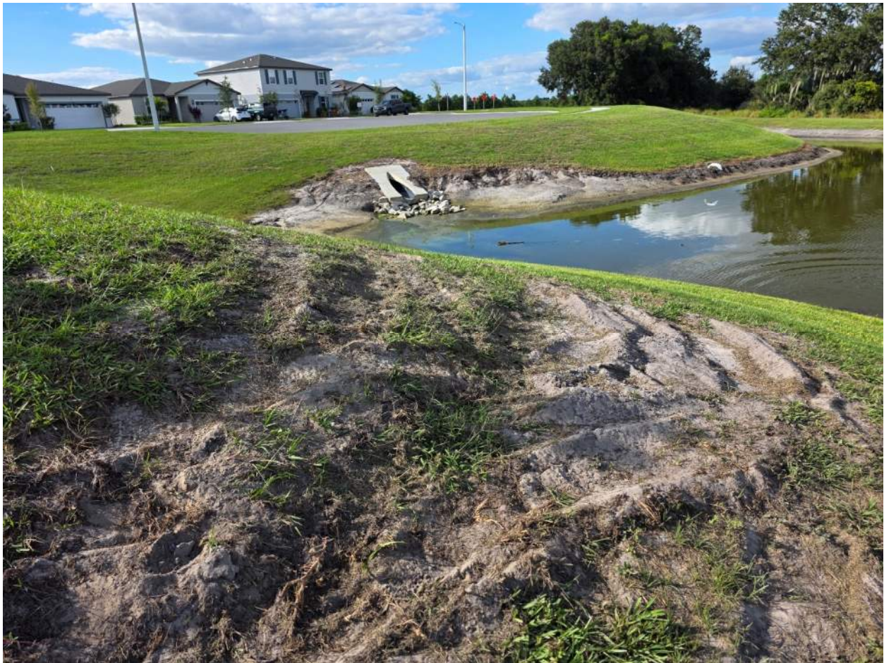
Figure 149. (Figure 149,151-152) Soil eroded around MES, restore grade and add sod.
