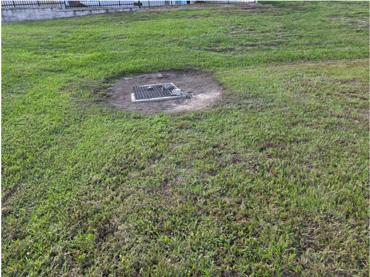
Figure 132. Area around control structure lacs vegetative cover, restore grade and sod around structure. Area should be mowed, not sprayed.
