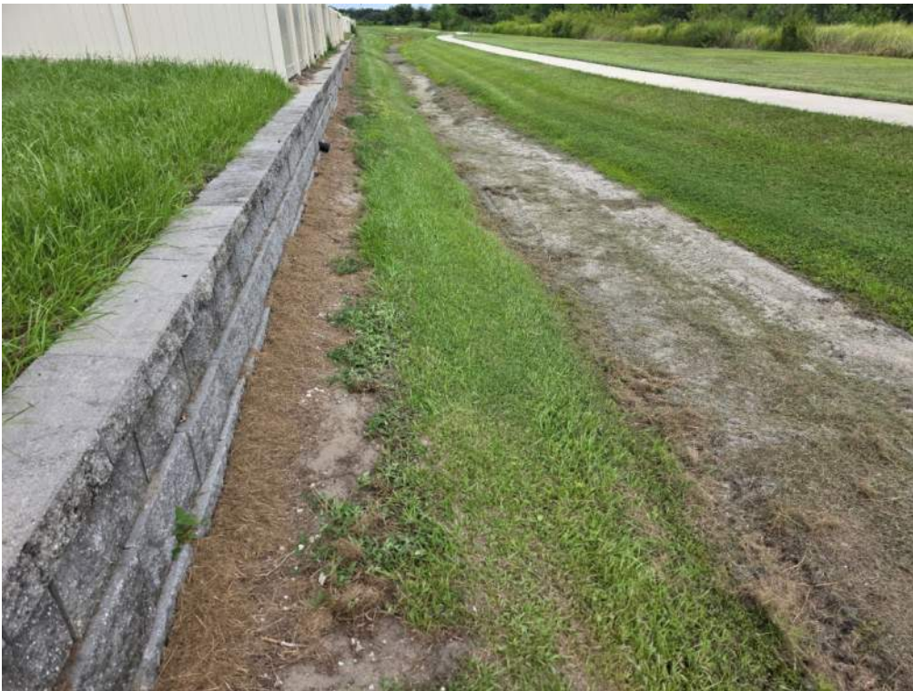
Figure 50. Large patch is bare of vegetation along bank. Add sod and monitor.
