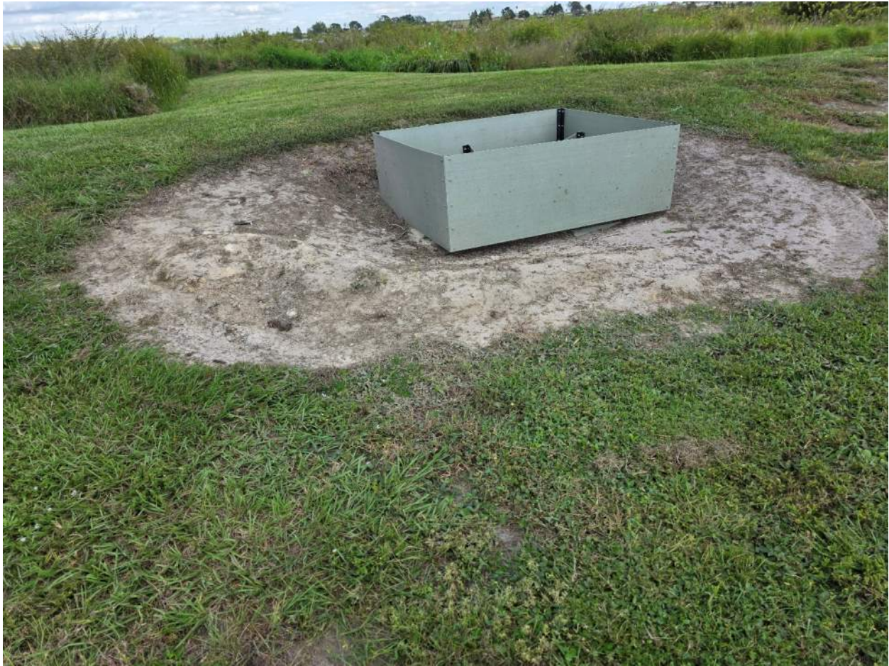
Figure 123. (Figure 123-125) Area around control structure lacs vegetative cover, restore grade and sod around structure. Area should be mowed, not sprayed.
