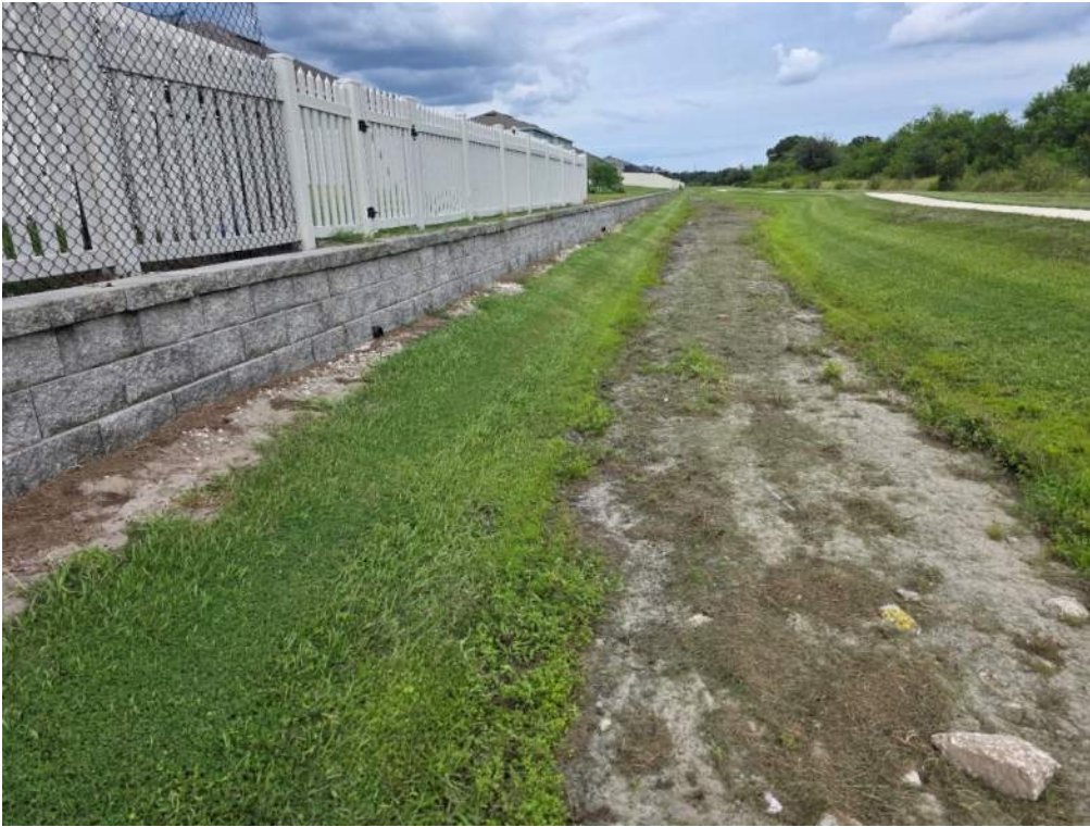
Figure 43. Large patch is bare of vegetation along bank. Add sod and monitor.
