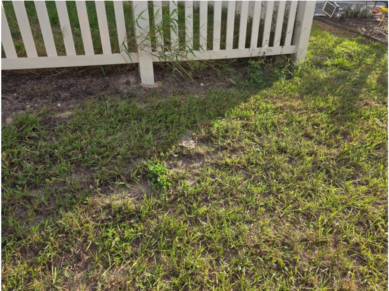
Figure 182. (Figure 182-186) Area lacks vegetative cover, fence post support exposed, reduce herbicide spraying, restore cover, and sod
