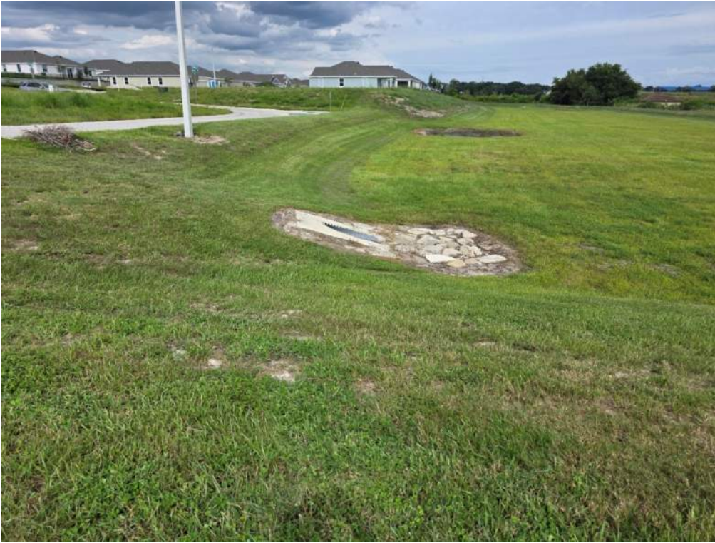
Figure 77. Loss of vegetative cover around MES. Add sod to restore cover.
