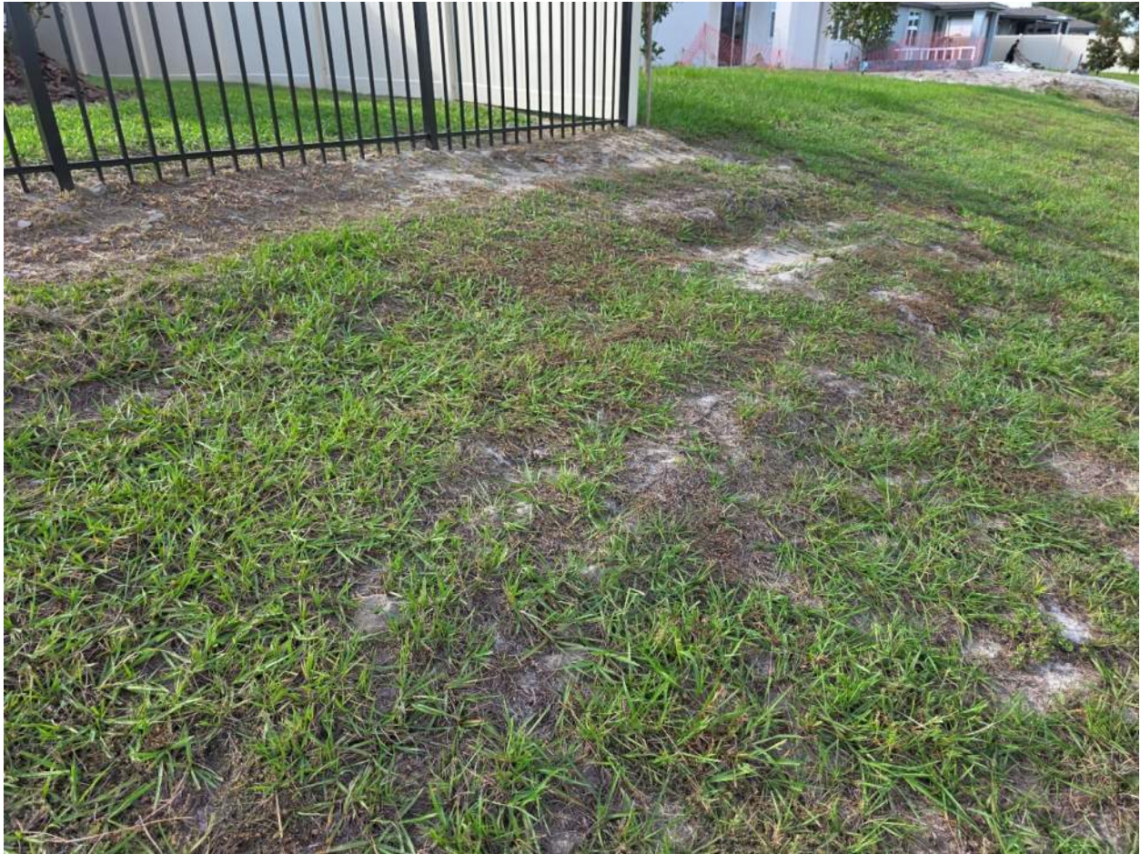
Figure 133. (Figure 133-137) Area lacks vegetative cover, fence post support exposed, reduce herbicide spraying, restore cover, and sod
