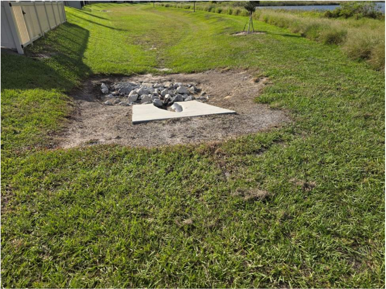
Figure 158. (Figure 158-159) Area around MES lacks vegetative cover, restore grade, sod and monitor
