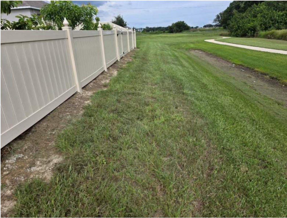
Figure 73. Large patch is bare of vegetation along bank. Add sod and monitor.
