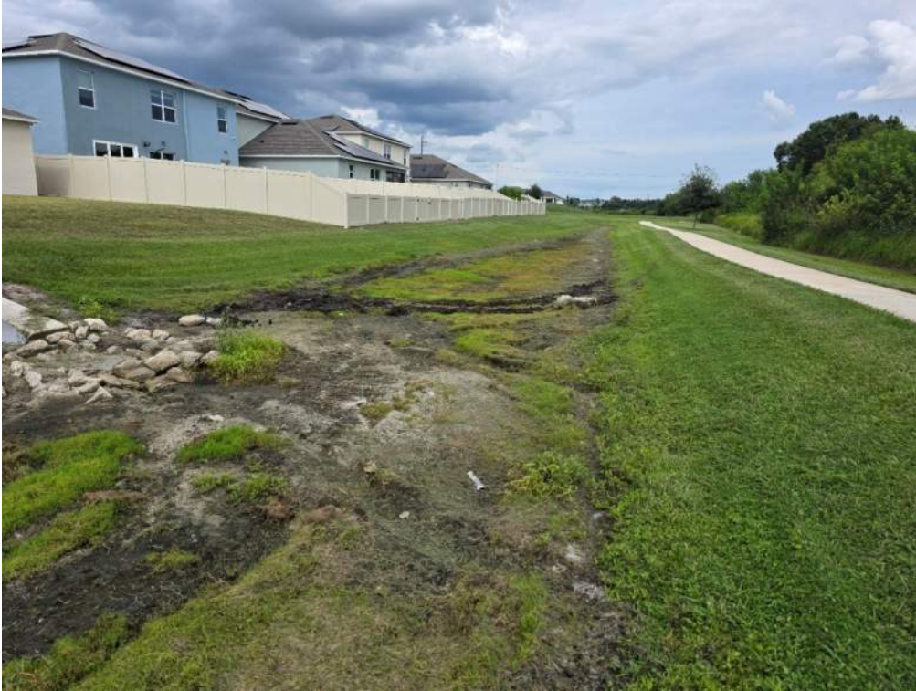
Figure 63. Baseline photo, bottom of pond. No action needed. Deep cuts in soil due to vehicles driving through pond.
