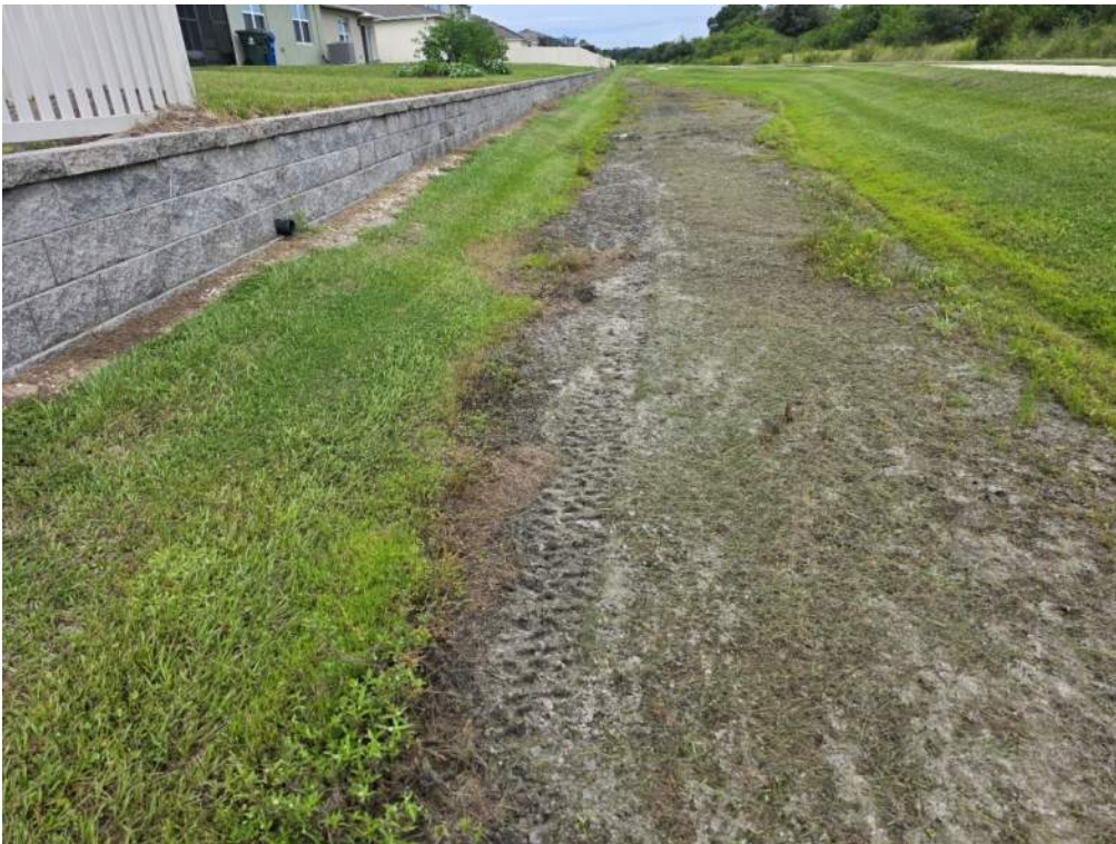
Figure 44. Large patch is bare of vegetation along bank. Add sod and monitor.
