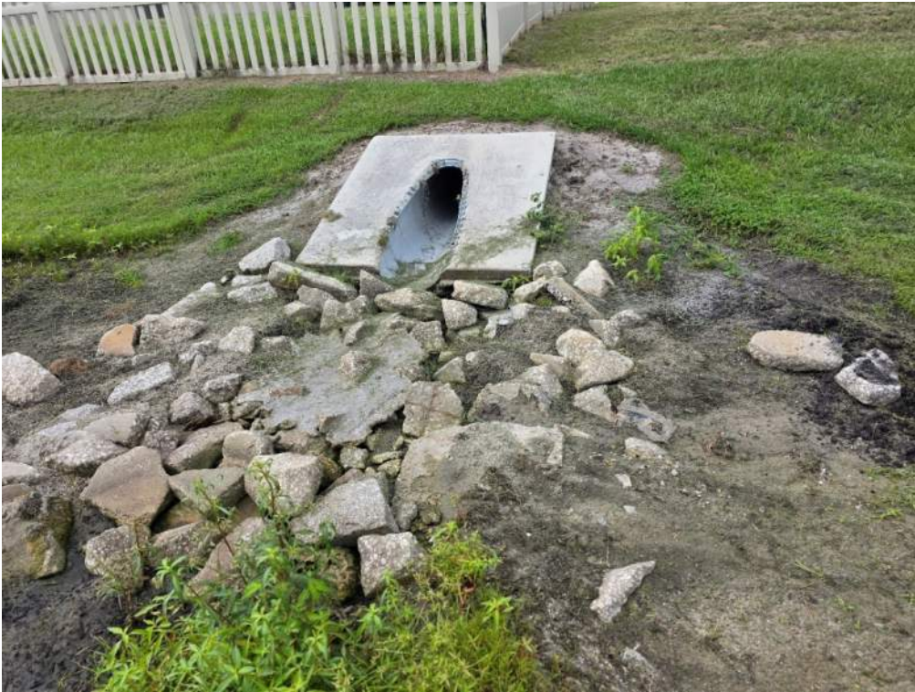
Figure 65. Area around and particularly below MES lacks vegetative cover and soil. Add soil to restore grade and sod. Rearrange riprap after grade restoration and monitor.
