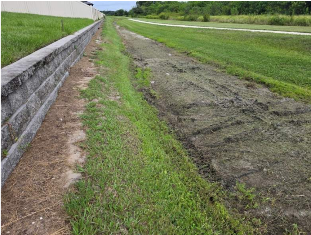
Figure 48. Large patch is bare of vegetation along bank. Add sod and monitor.
