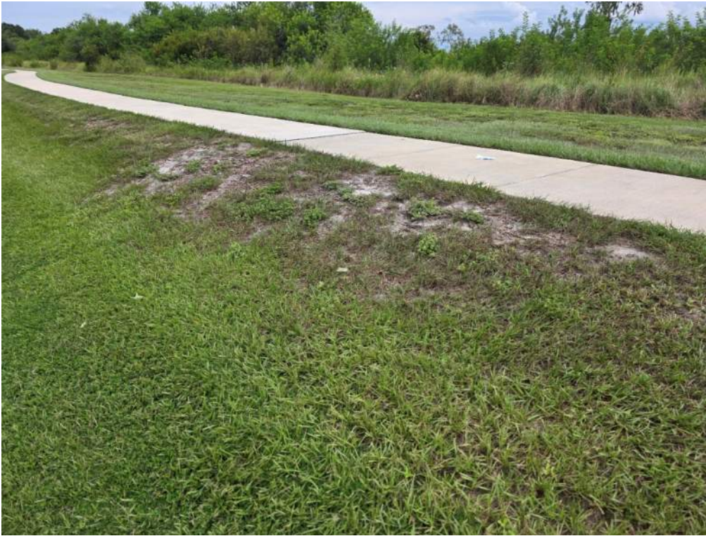
Figure 41. Vegetation thinning and erosion near sidewalk. Add sod and monitor.
