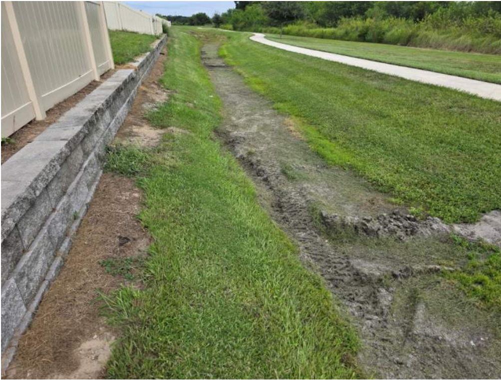
Figure 53. Large patch is bare of vegetation along bank. Add sod and monitor.
