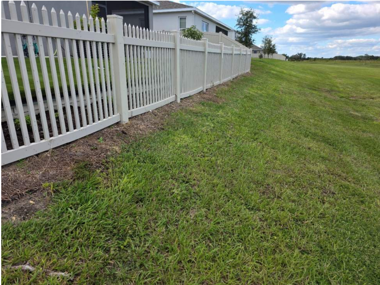
Figure 80. (Figure 80-82) Area lacks vegetative cover, fence post support exposed, reduce herbicide spraying, restore cover, and sod
