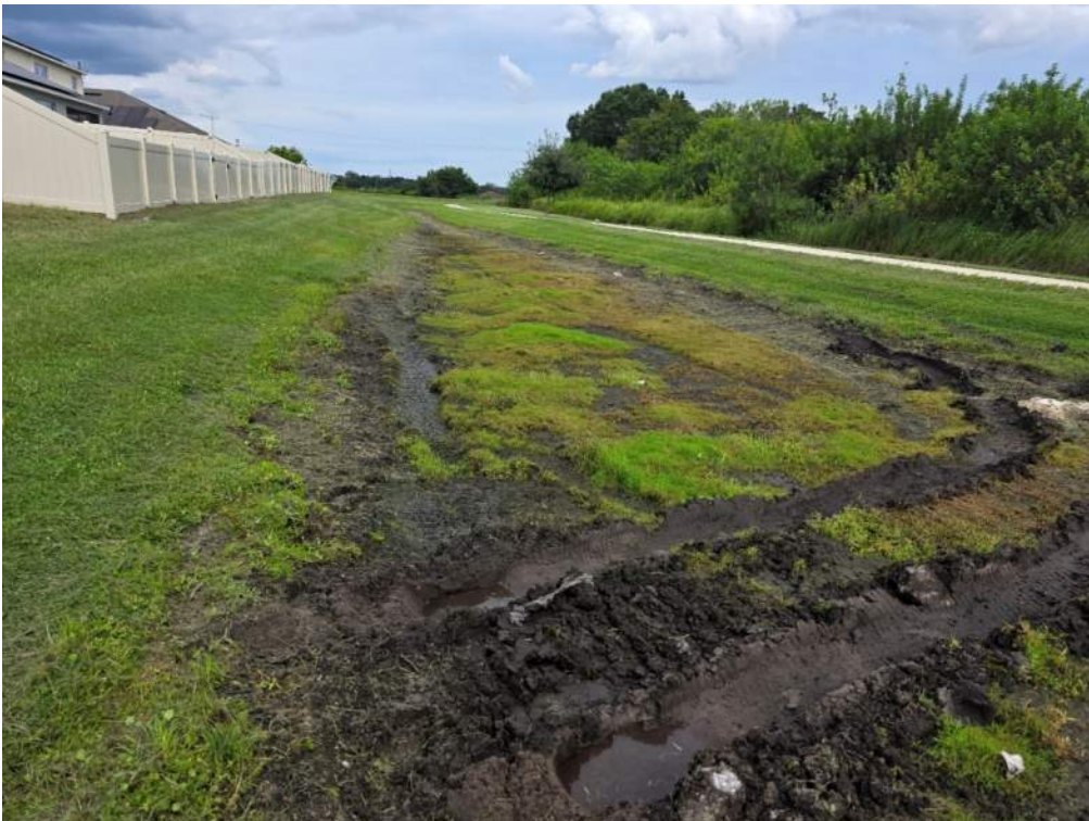
Figure 68. Baseline photo, bottom of pond. No action needed. Deep cuts in soil due to vehicles driving through pond.
