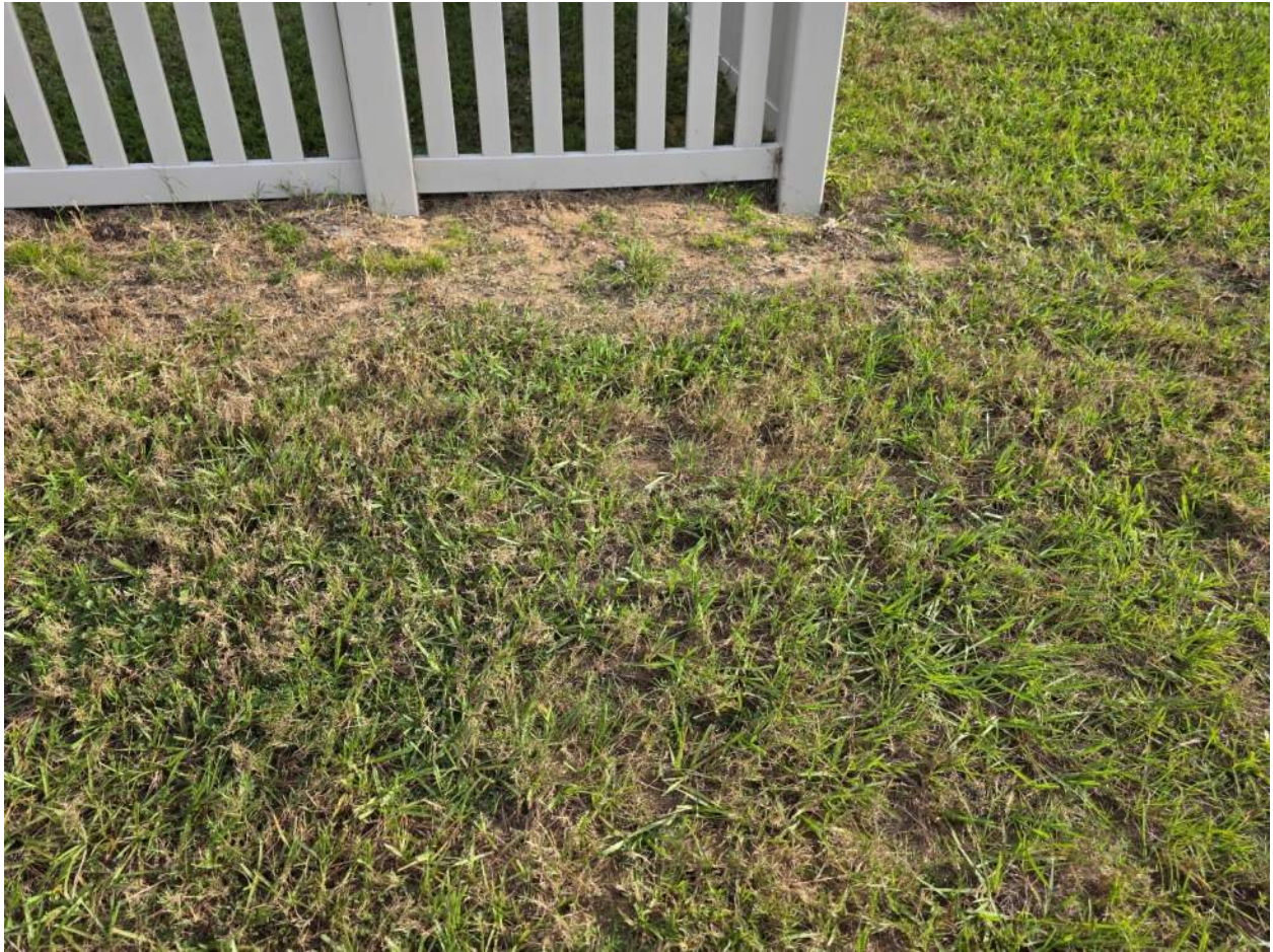
Figure 191. (Figure 191-197) Area lacks vegetative cover, fence post support exposed, reduce herbicide spraying, restore cover, and sod
