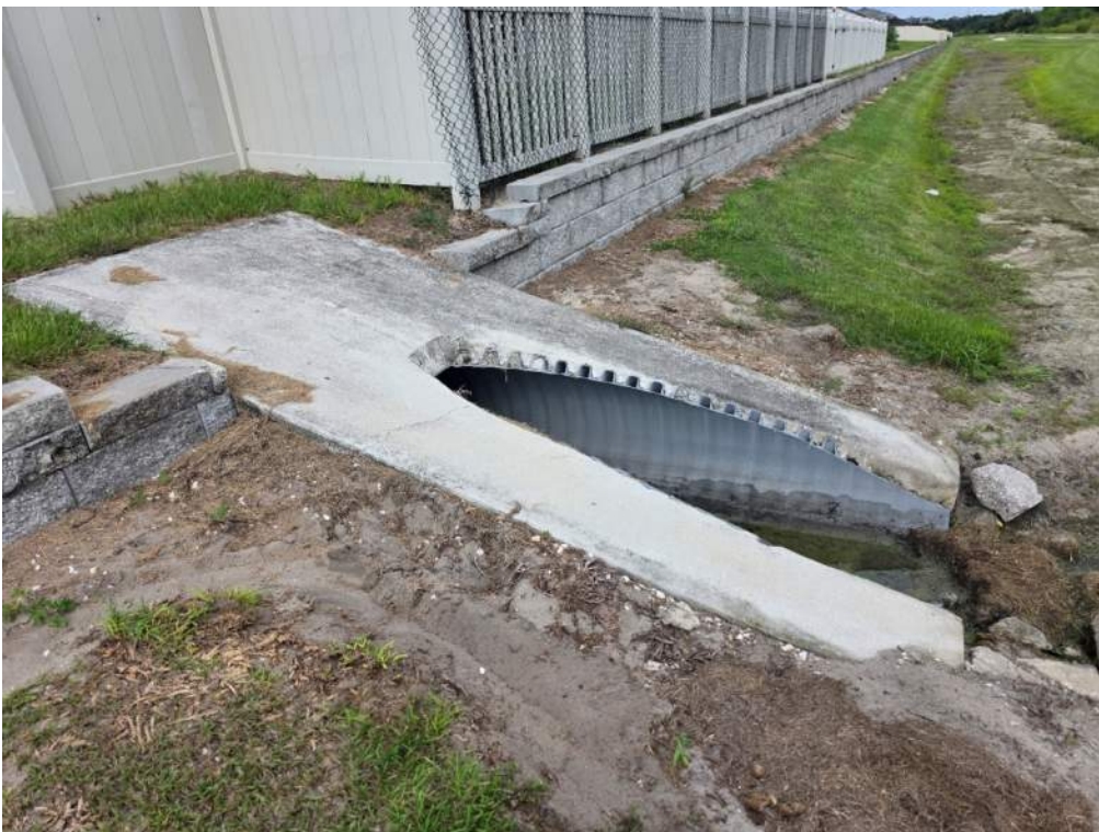
Figure 38. Complete lack of vegetation near MES and retaining wall containing yard drains. Install new sod along structure and wall to prevent further erosion and sedimentation.
