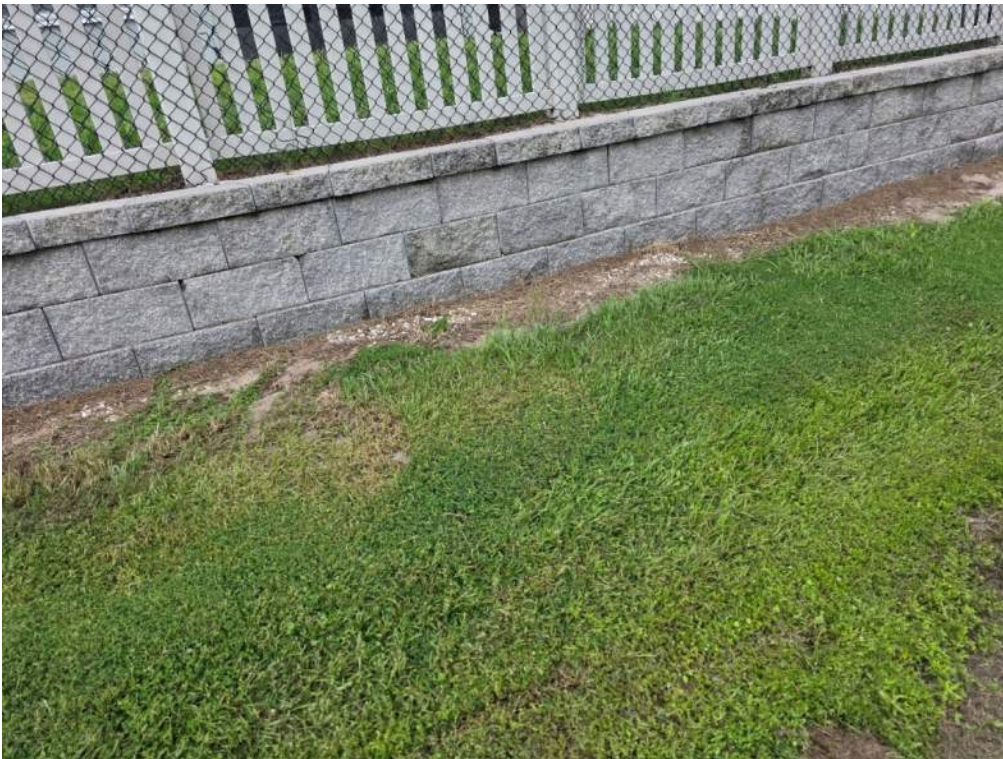
Figure 42. Large patch is bare of vegetation along bank. Add sod and monitor.
