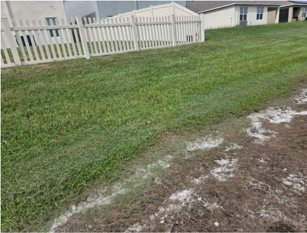
Figure 31. Large patch is bare of vegetation along bank. Add sod and monitor.
