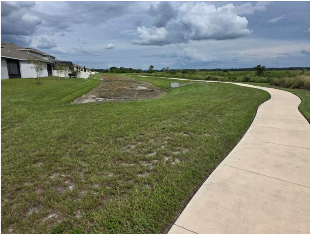
Figure 2. Drainage area lacks sufficient vegetative cover. Add sod along slope and monitor.
