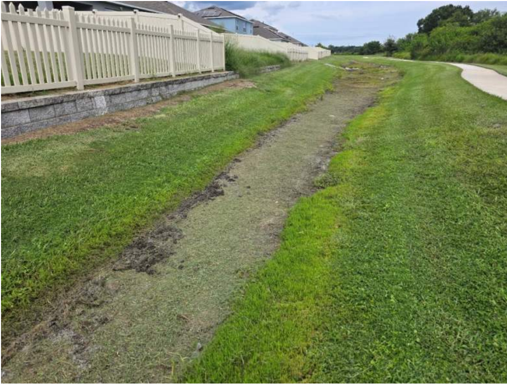
Figure 57. Large patch is bare of vegetation along bank. Add sod and monitor.
