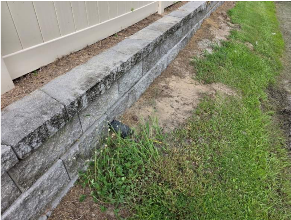
Figure 54. Yard drain downturned into soil. Reorient for proper drainage.
