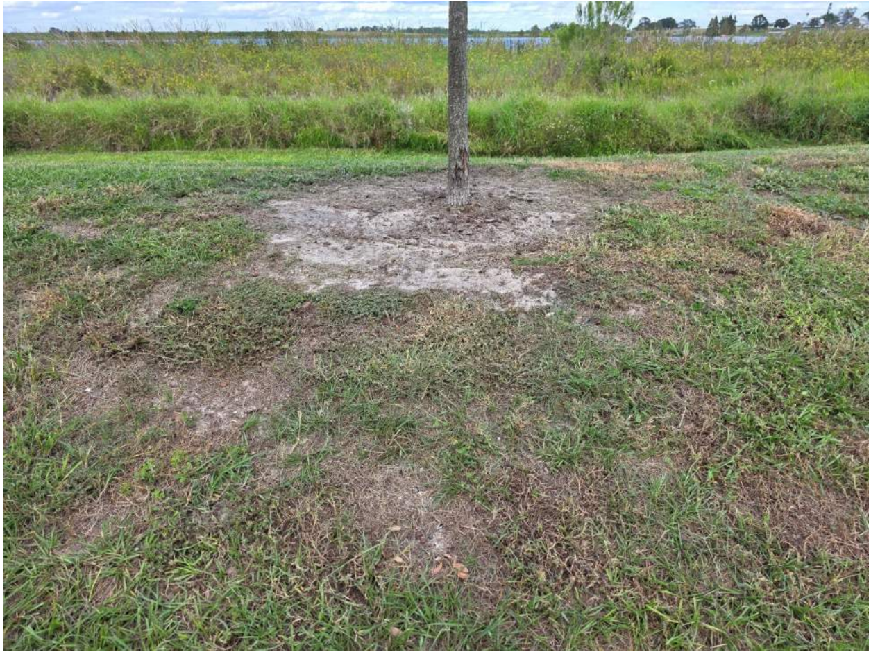
Figure 100. Vegetative cover reduced, reduce spraying, monitor
