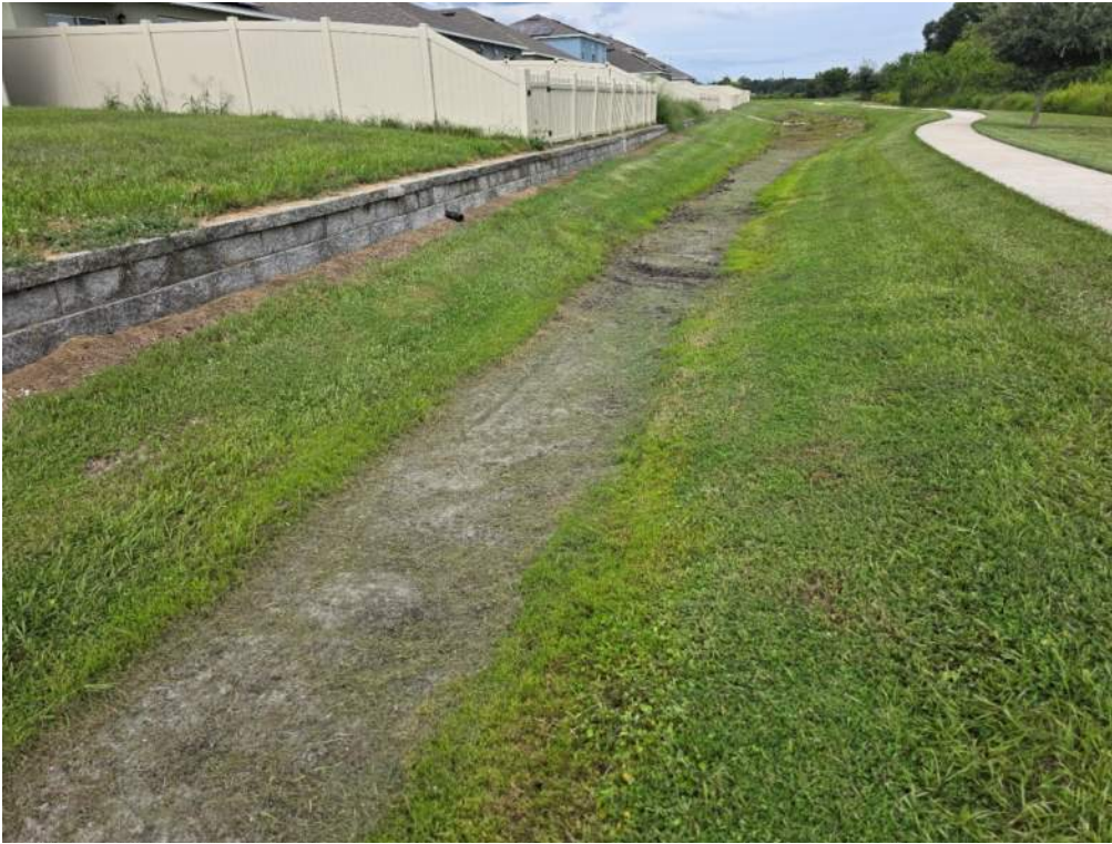
Figure 55. Large patch is bare of vegetation along bank. Add sod and monitor.
