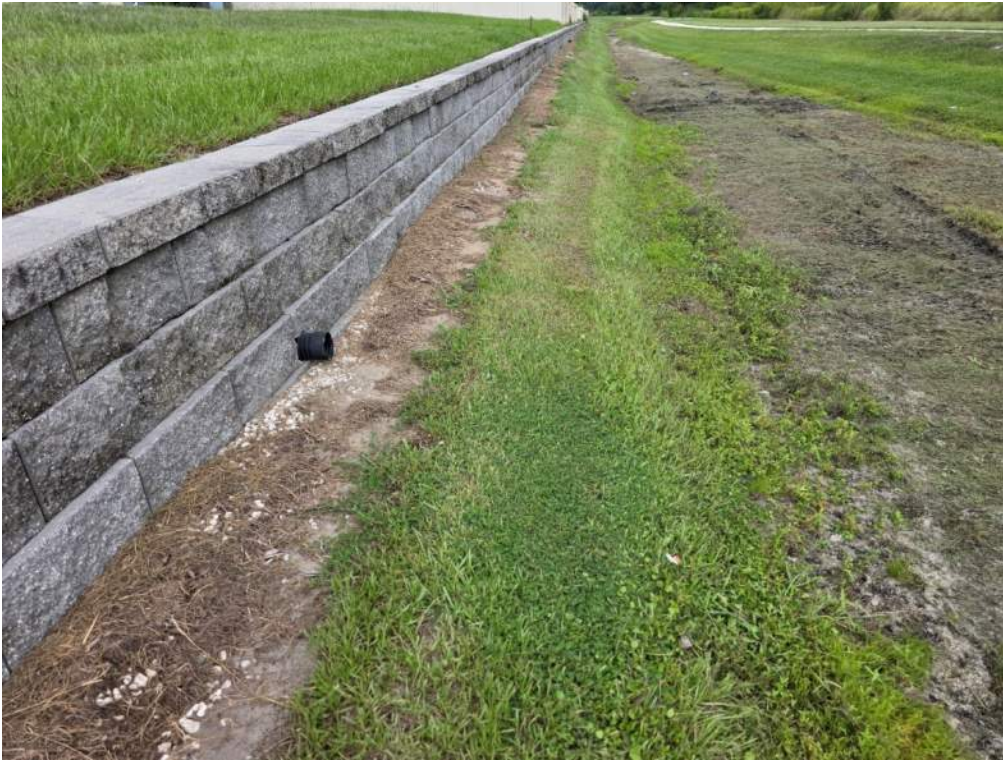
Figure 47. Large patch is bare of vegetation along bank. Add sod and monitor.
