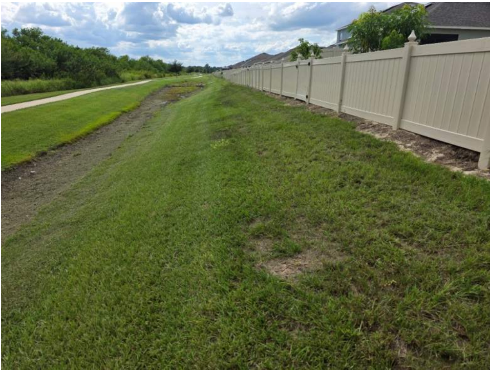
Figure 76. Small patch is bare of vegetation along bank. Add sod and monitor.
