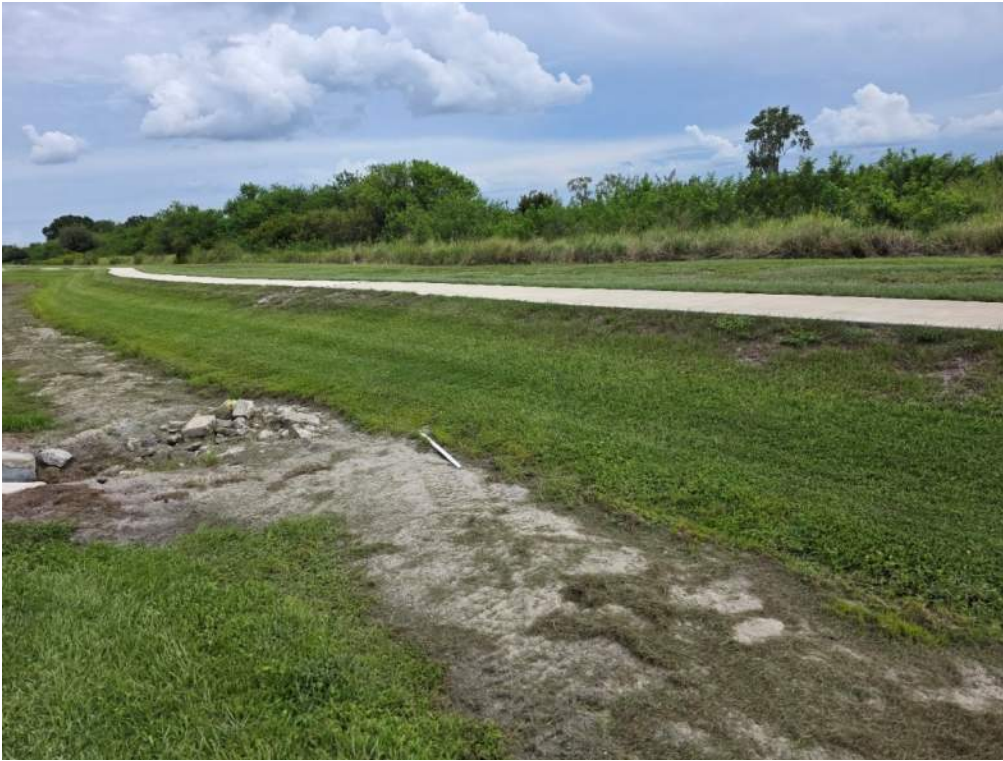
Figure 37. Vegetation thinning and erosion near sidewalk. Add sod and monitor.
