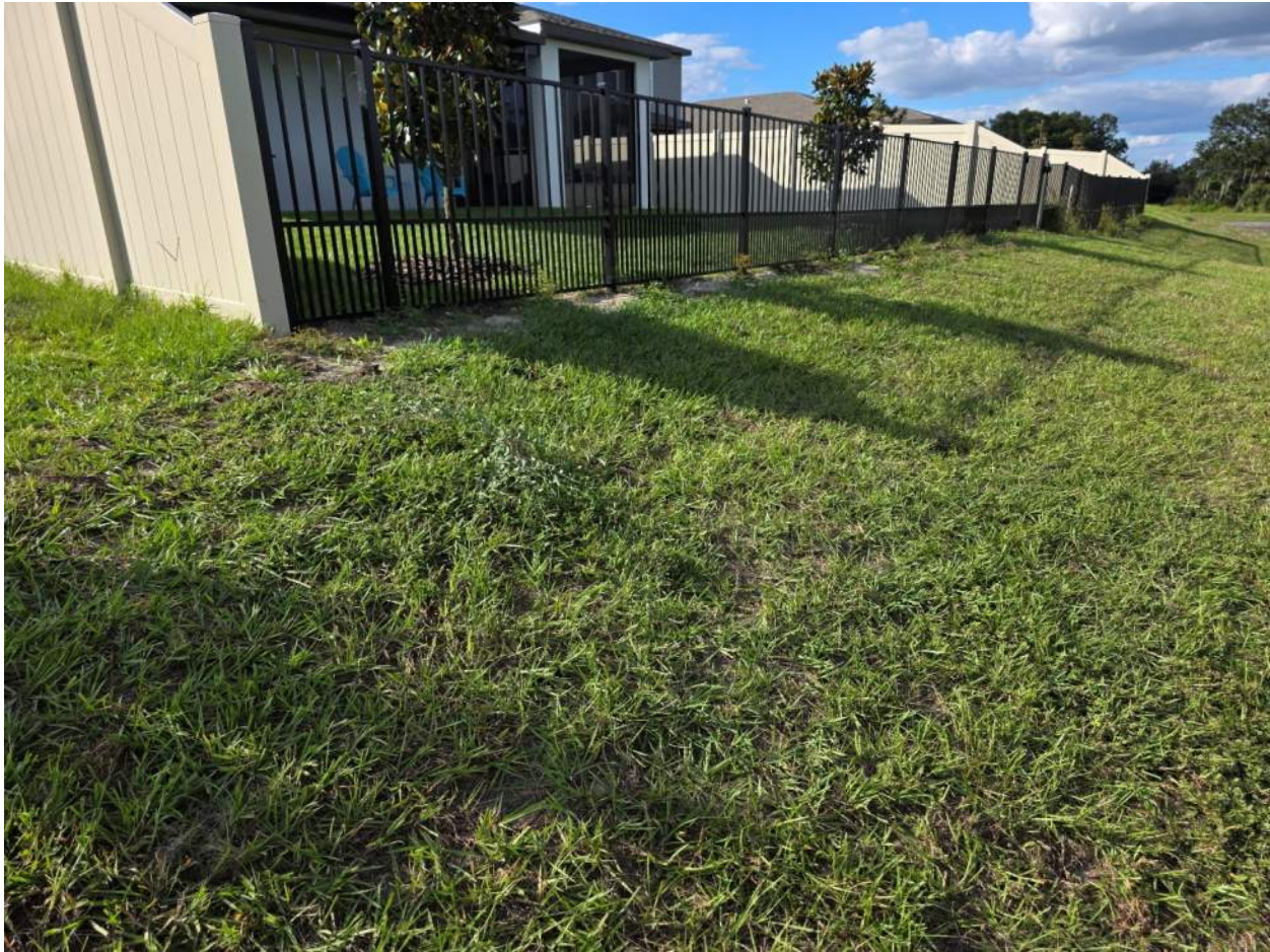
Figure 141. (Figure 141-145) Area lacks vegetative cover, fence post support exposed, reduce herbicide spraying, restore cover, and sod
