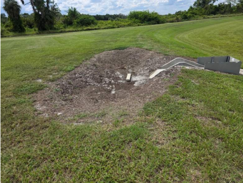
Figure 1. Drainage area lacks sufficient vegetative cover. Add sod along slope and monitor.
