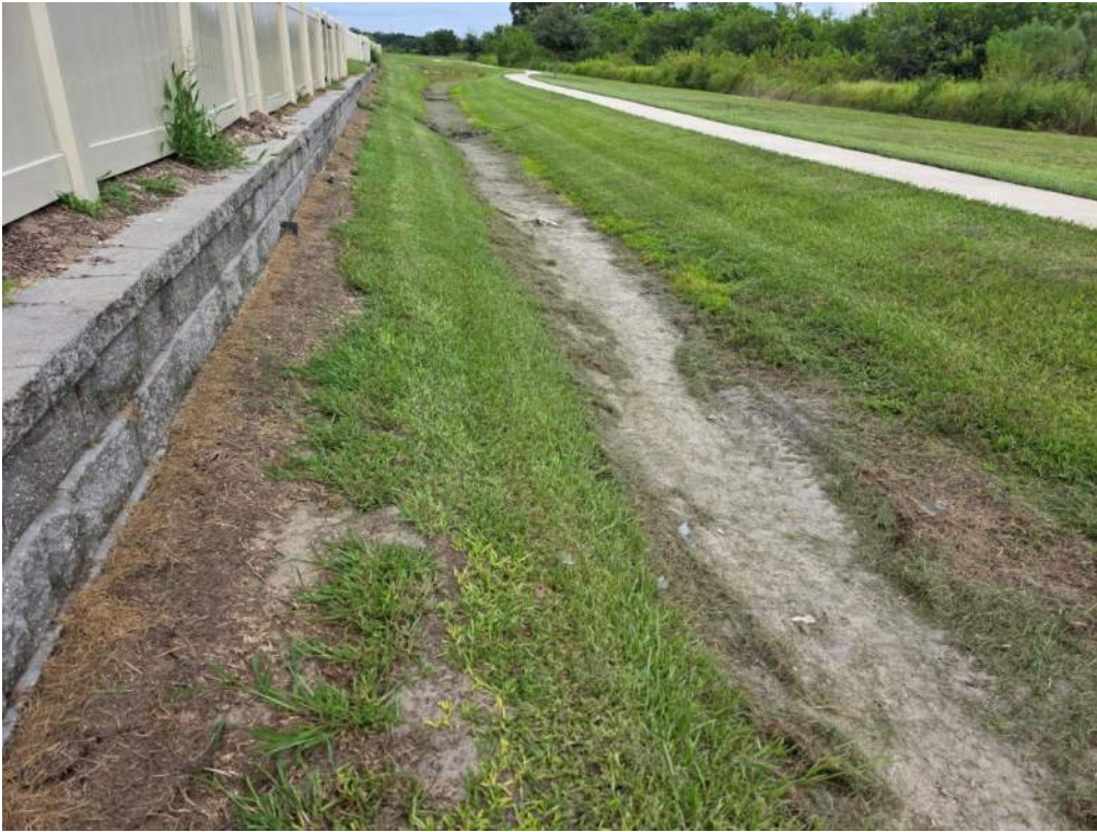
Figure 51. Large patch is bare of vegetation along bank. Add sod and monitor.
