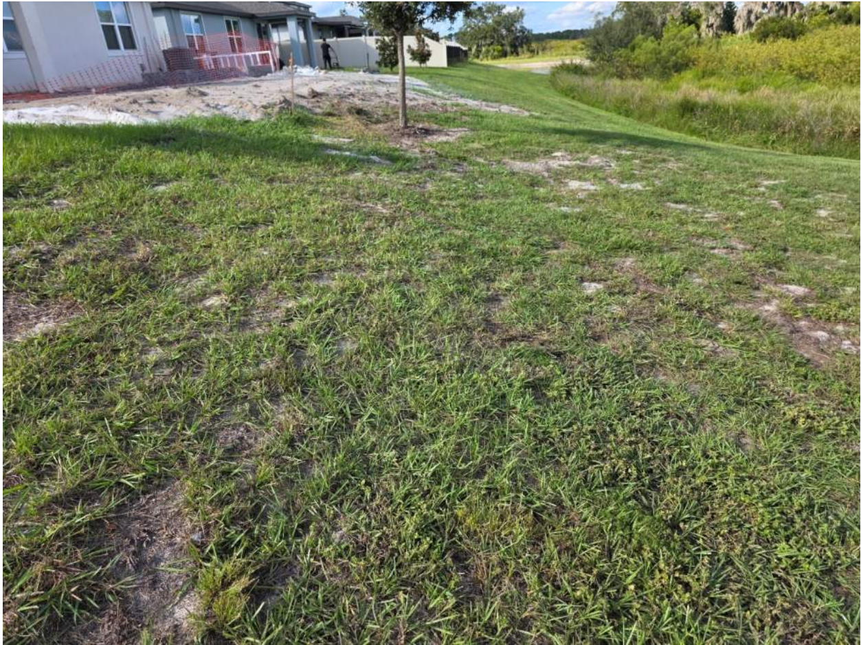
Figure 138. (Figure 138-140) Construction area lacks silt fencing, make contact with resident and ensure runoff is not deposited or left in abutting wetland or CDD owned lands.
