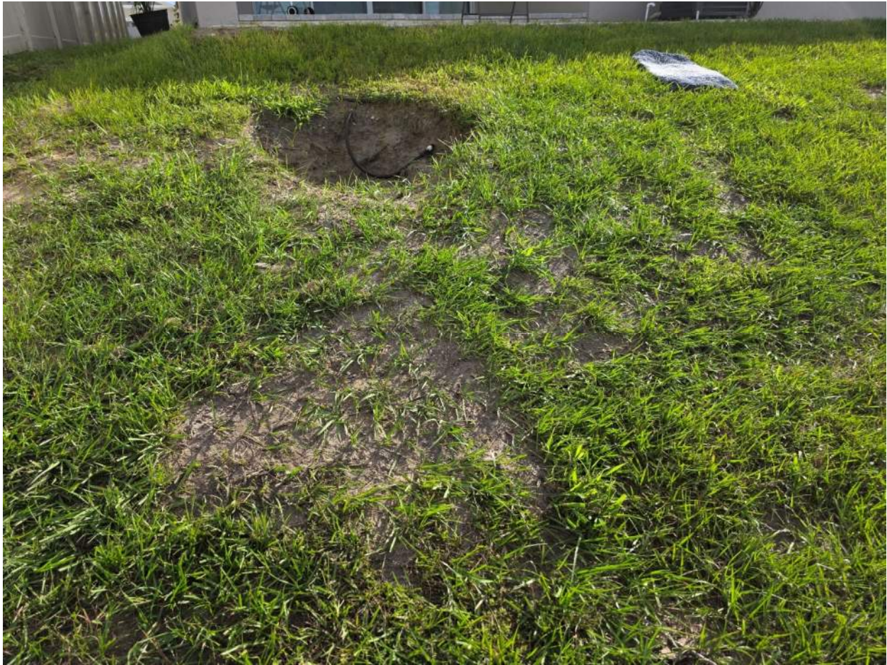
Figure 164. Resident's irrigation has caused a massive depression on their property which will affect drainage into the pond. Notify them to correct this by filling and sodding hole as well as fixing irrigation issue.
