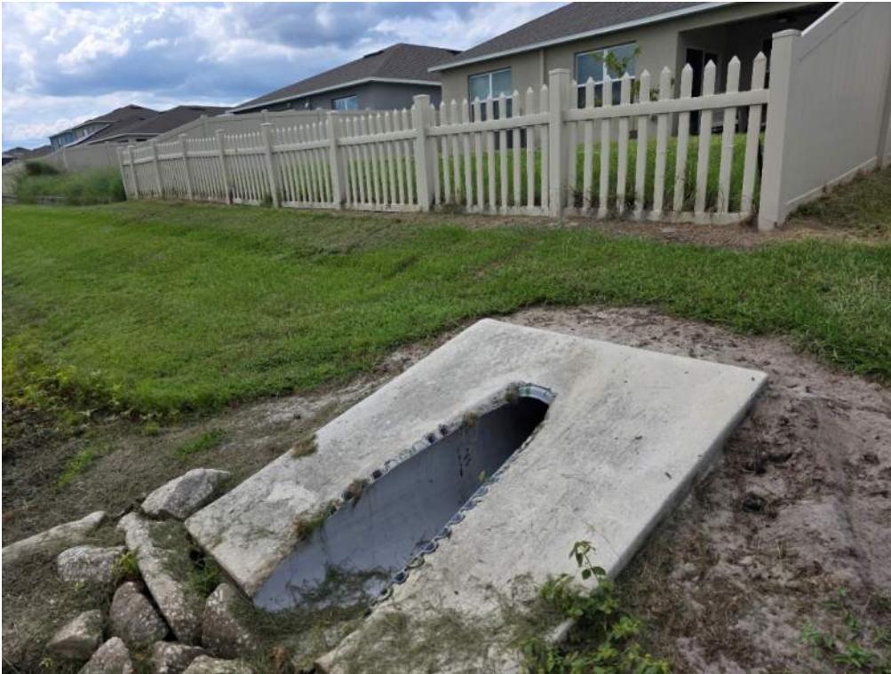
Figure 67. Area around and particularly below MES lacks vegetative cover and soil. Add soil to restore grade and sod. Rearrange riprap after grade restoration and monitor.
