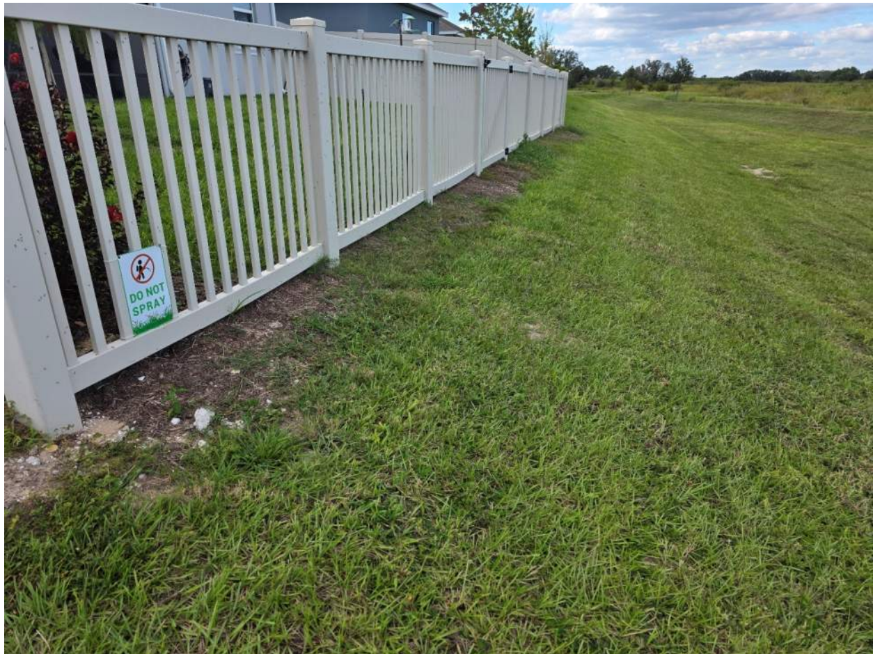
Figure 91. (Figure 91-96) Area lacks vegetative cover, fence post support exposed, reduce herbicide spraying, restore cover, and sod
