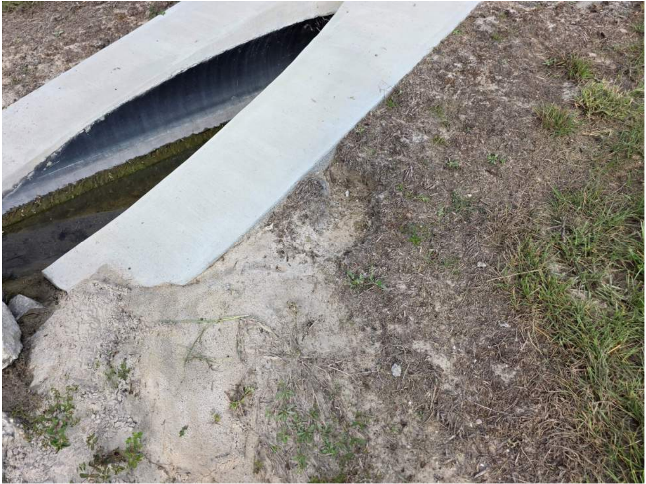
Figure 224. (Figure 224-225) Restore grade around MES and sod
